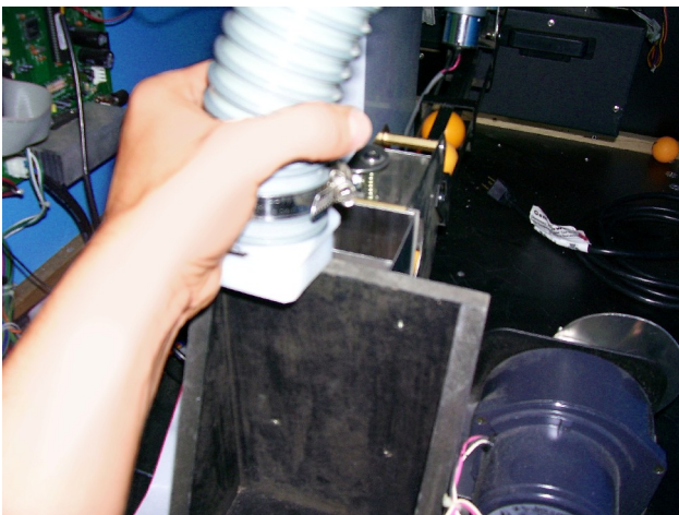
Replace Vent Pipe and attachment back into the Sending Main Frame
